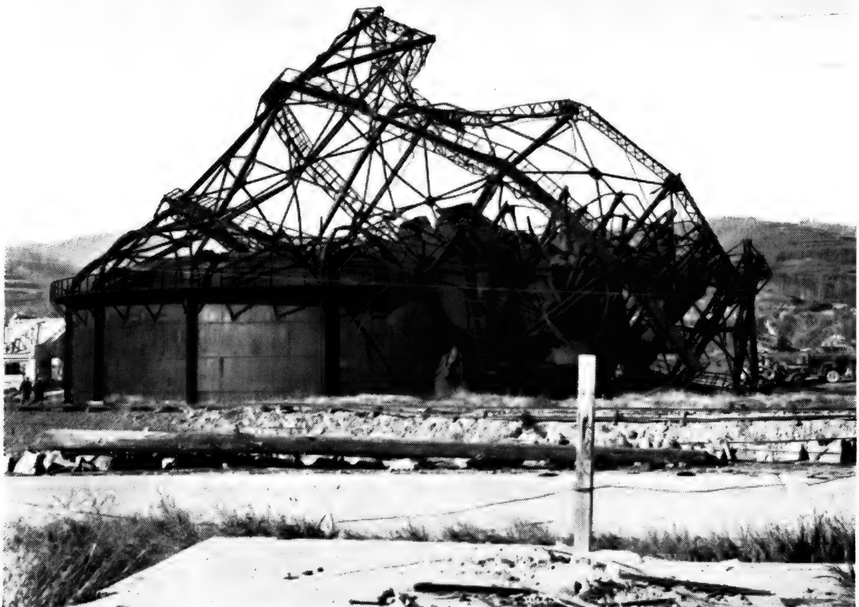
Photo No. 14. NAGASAKI. Blast effect on a gasholder \frac{1}{2} mile from centre of damage. Note the way in which the whole framework has been bent away from the explosion. See paragraph 43.
